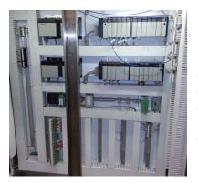
A new electrical room was constructed in the Disinfection Storage Building for the new Motor Control Center (MCC), the new PLC panel, and associated electrical equipment. A new PLC panel was installed along with all new instrumentation and field controls. All electrical and I&C components in the building were replaced.
